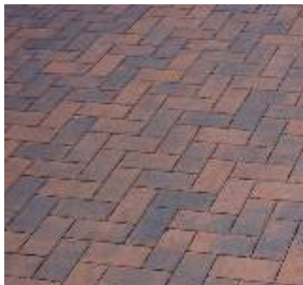
Concrete block paving
