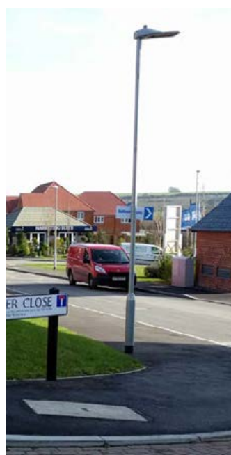
Lighting column to meet highway requirements
