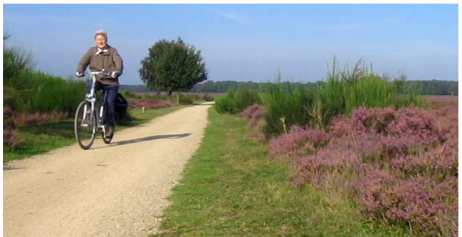
Self binding gravel cycle way
